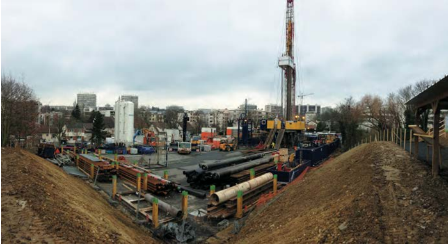
Figure 1.12 Drilling pad for a geothermal doublet near Paris (source: CFG).
