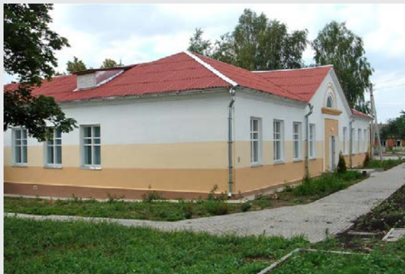
FIGURE 1. The Bragin Museum after renovation (photo: J. Lochar).
