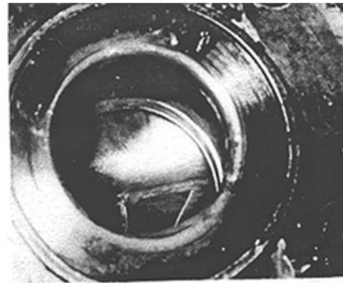
Circuit section with the use of CTS (after introduction of cleaning system)
